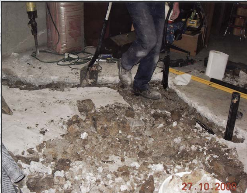
Breaking concrete for new drain line...
