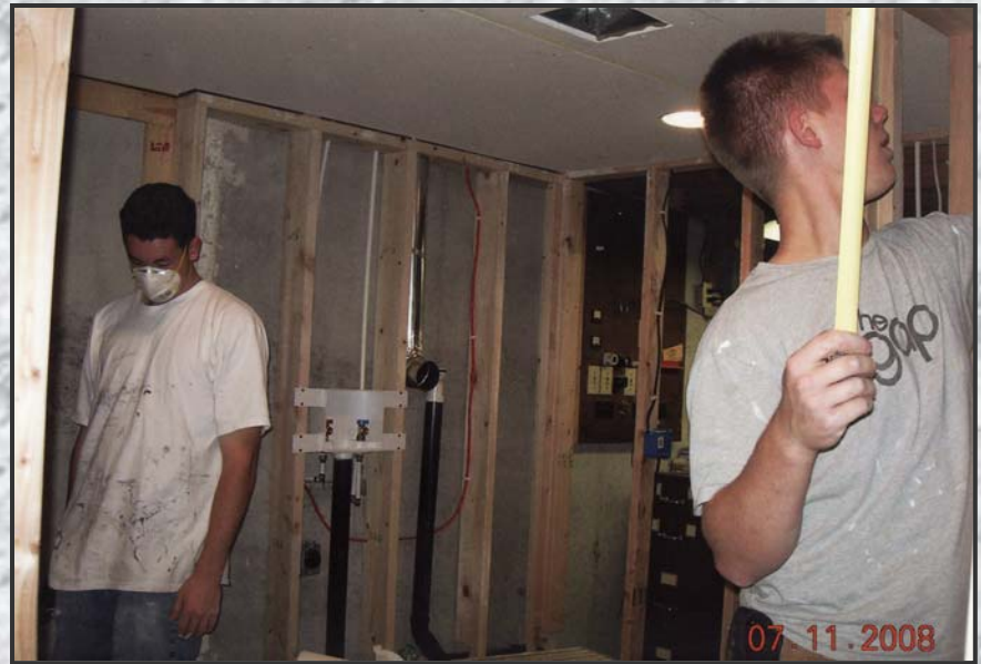
Framing & Hanging new sheetrock...
