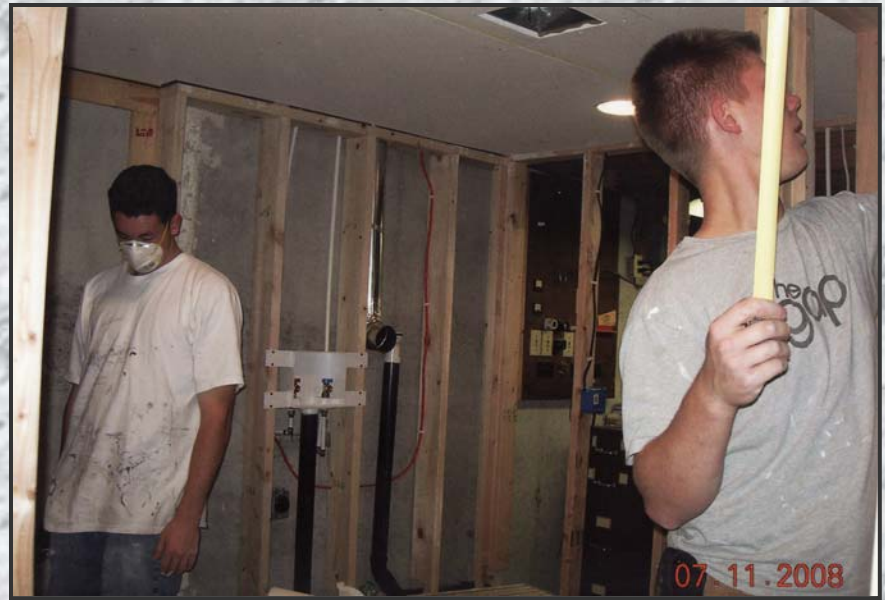
Framing & Hanging new sheetrock...
