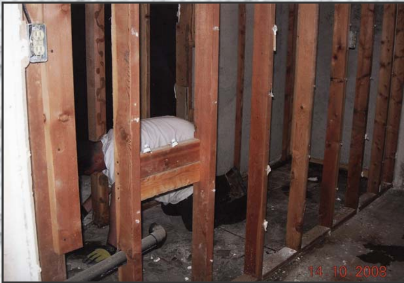
Bathroom before expansion...
