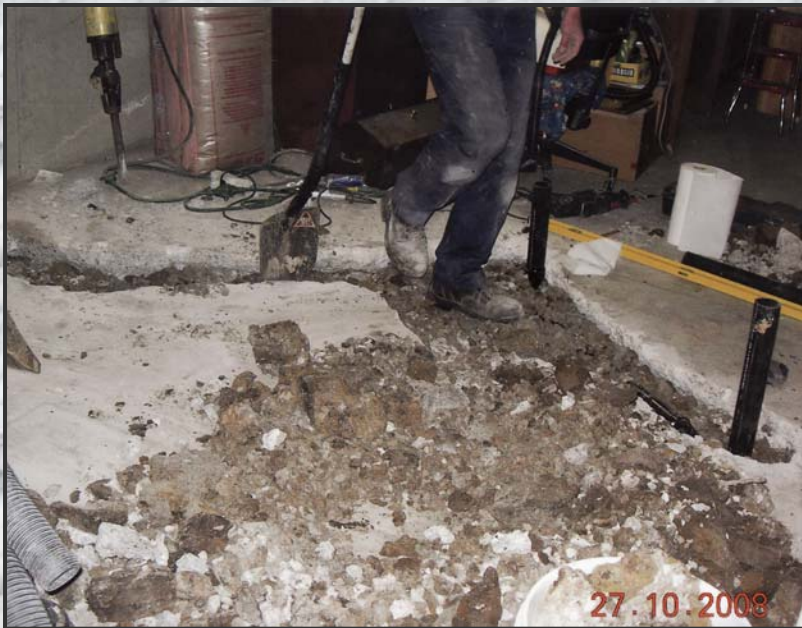
Breaking concrete for new drain line...
